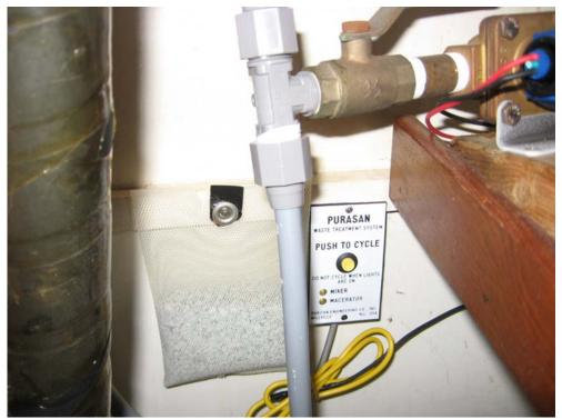
Picture #5 Purasan "push to cycle switch" under the sink in the aft head.
